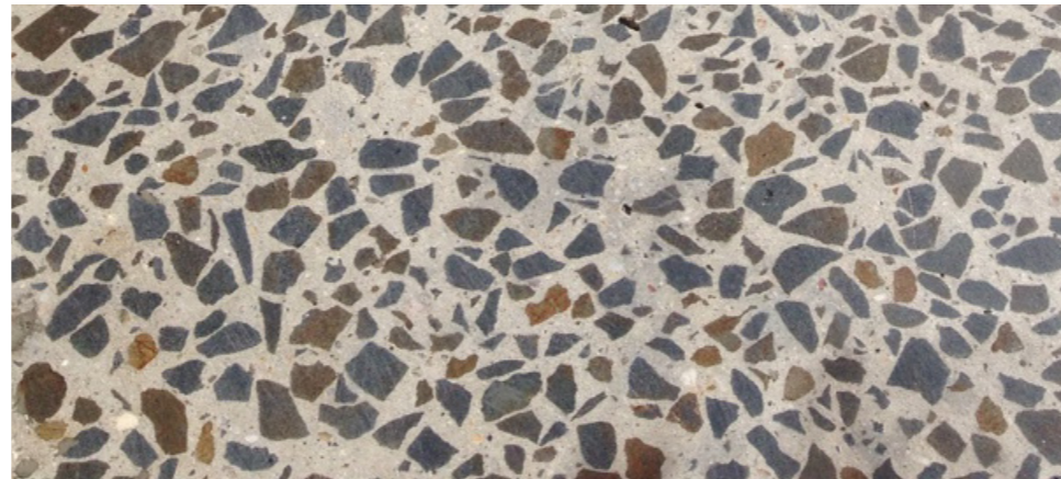
A concrete pathway after honing
