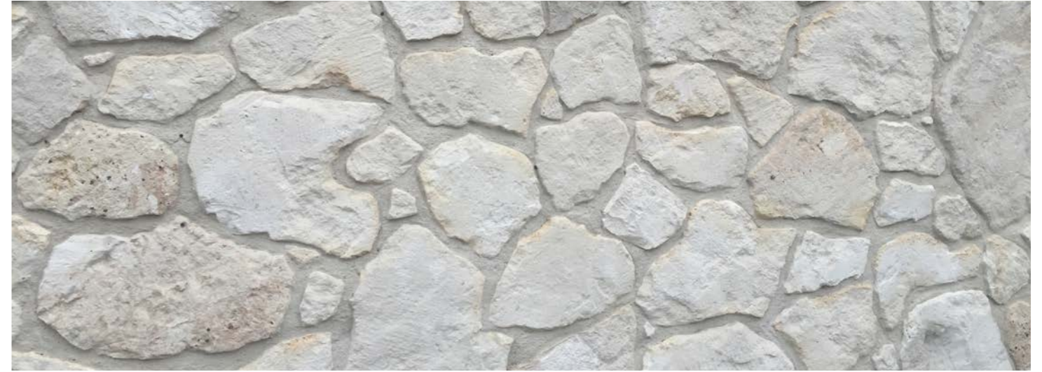
Fig 27: Feature stone walls
