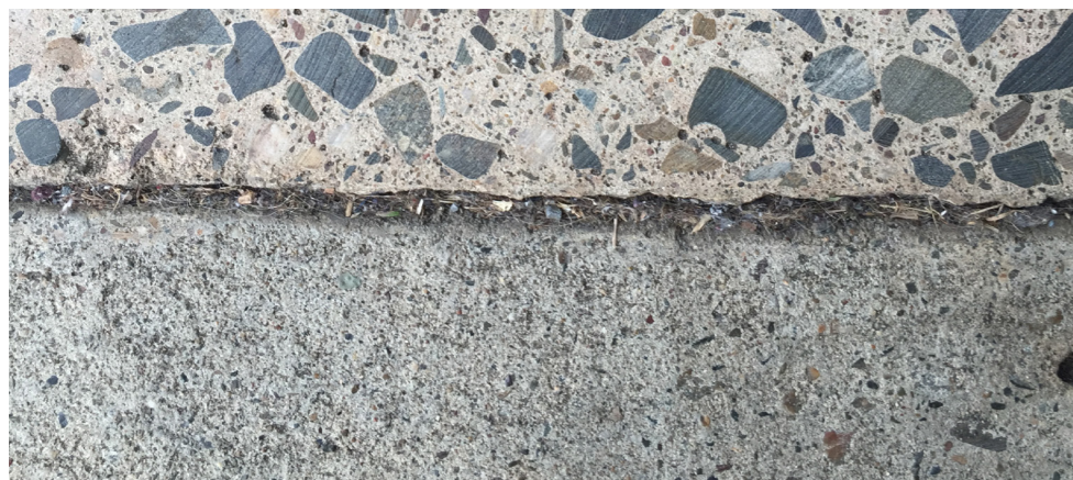
A before and after concrete honed path
